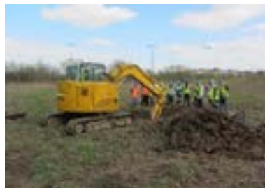
b) Trial Pit Excavation
