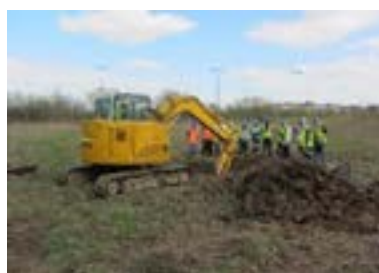
b) Trial Pit Excavation
